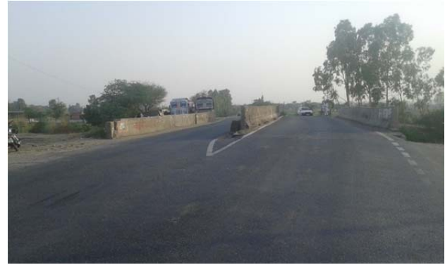
Fig. 5 Black spot on Rohat River Bridge
